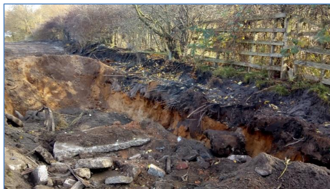
Excavations taking place at time of initial investigation
